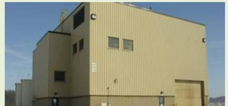
Wastewater Treatment Plant
