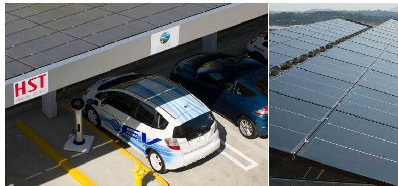
Honda CIGS thin-film solar cells installed on the roof and carport of Honda Performance Development in Santa Clarita, California.
