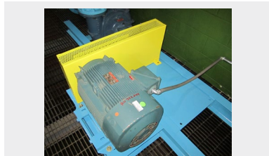
Micro-hydropower generation system at the Marysville, Ohio auto plant.
